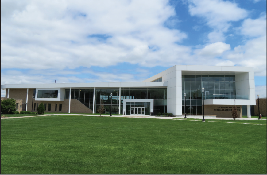
The Marlene and Joe Toot Global Learning Center at Walsh University Tile Installation by Youngstown Tile & Terrazzo - Canfield, OH
